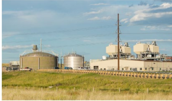
Figure 05-4 Cheyenne Prairie Generating Station Combined Cycle CT
