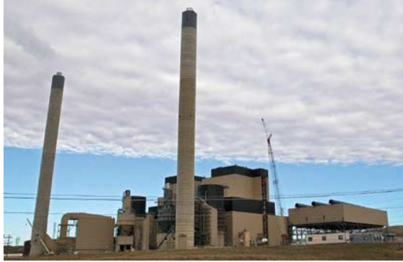
Figure 05-2 Wygen II and Wygen III Generation Facility
