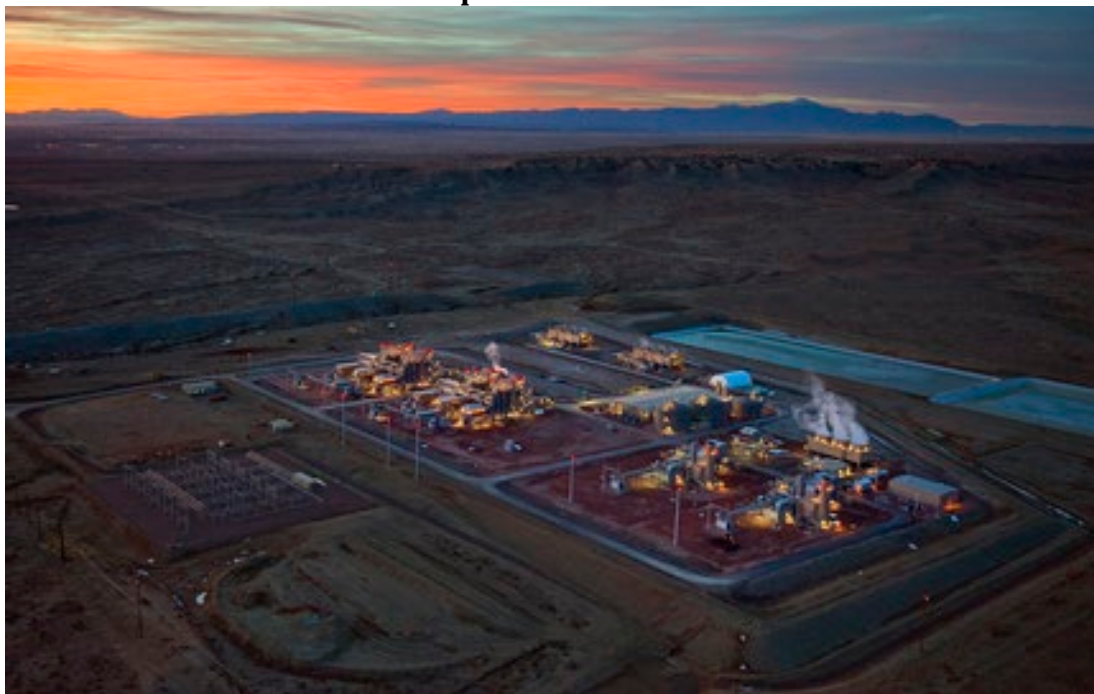
Figure 5-1 Pueblo Airport Generation Station
