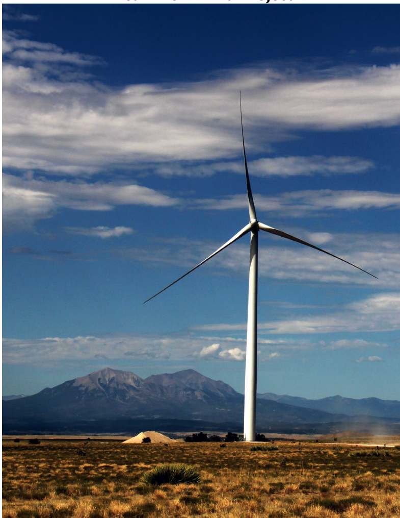
Figure 5-3 Peak View Wind Project
