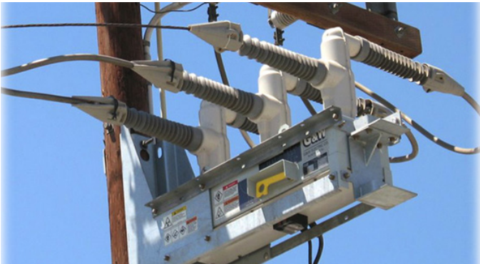
Figure 21: Example – Distribution line recloser.
